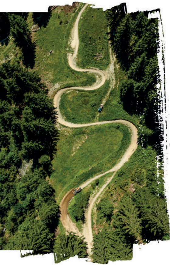
The powerful D501 shaping a mountain bike trail.
